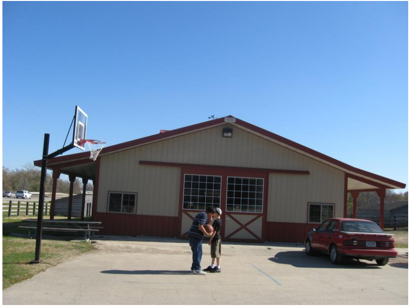
Horse Barn and Basketball Court
